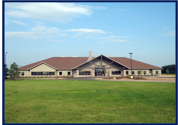
The Life Center Completed 2008 Funded by Gift From Anonymous Donor and Others
