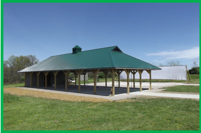
Naomi Dempsey Accessible Archery Shelter Completed 2017 Funded by the All Life Foundation
