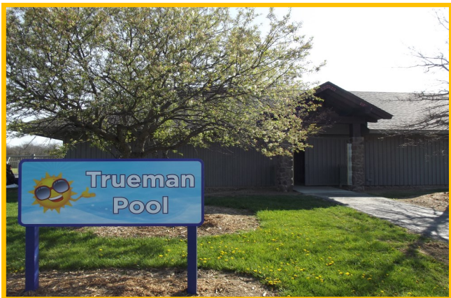
Trueman Pool House Renovation & Addition—Completed 2016 Major Funders Muirfield Invitational Golf, All Life Foundation & Anonymous
