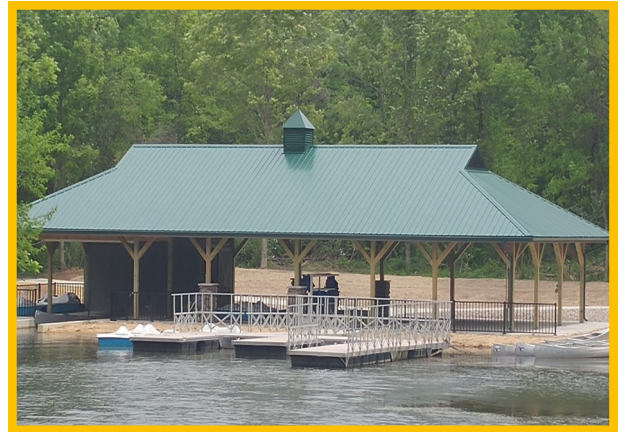
The Ginni D. Ragan, John, Kevin and Arin McNamara Families Boat House and Accessible Canoe Launch Completed 2019 Funded by the All Life Foundation
