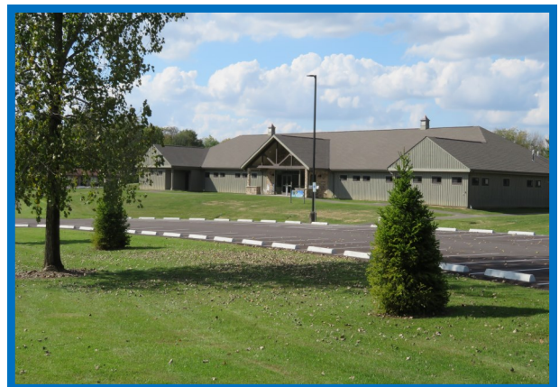
The Greif Retreat House Completed 2018 Major Funders Greif, Inc. & All Life Foundation
