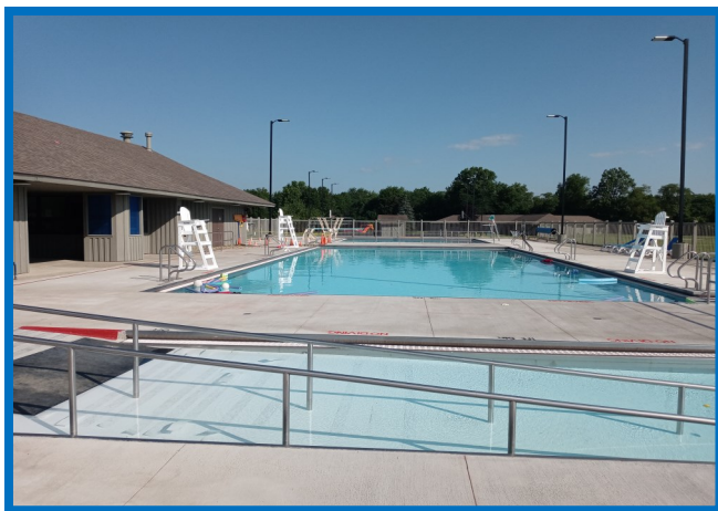
The Trueman Pool Completed 2022 Funded By The All Life Foundation
